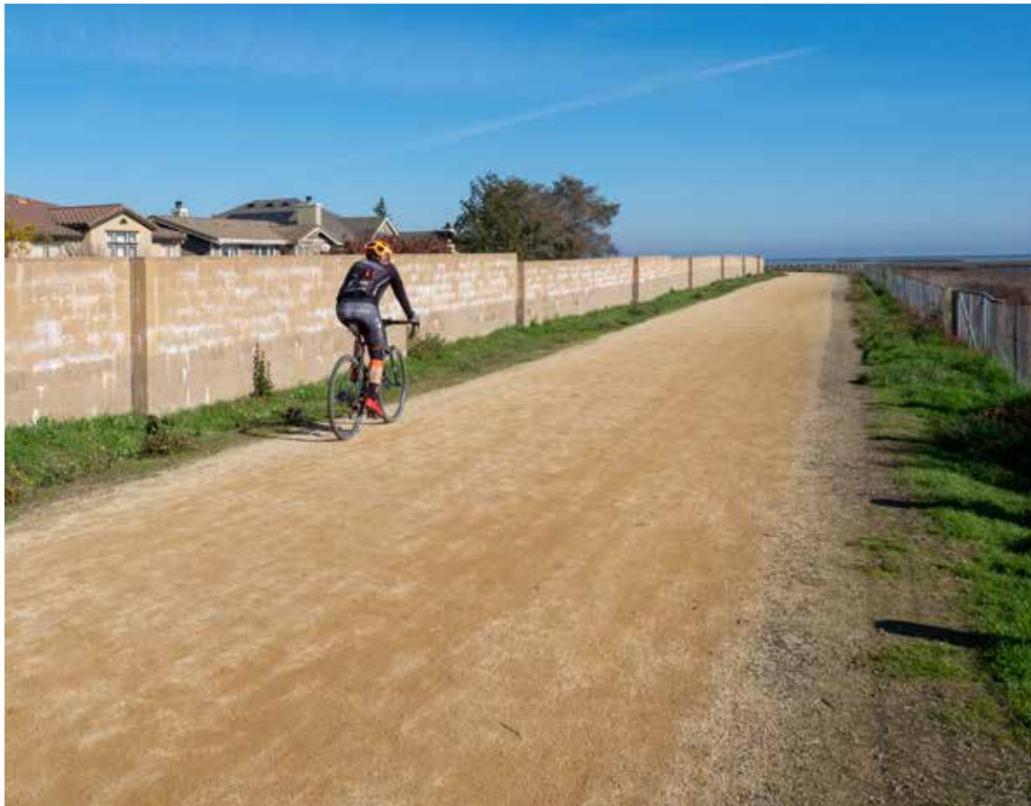
A flood wall adjacent to the Bay Trail near Hamilton Wetlands in Marin County (photo by Shira Bezalel, SFEI)
