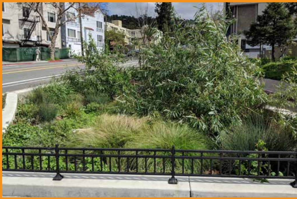
Stormwater detention basin with native plants in Berkeley, CA. Photograph by Robin Grossinger, SFEL.
