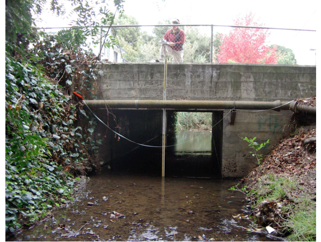
A) View looking upstream at the Curtiss Street bridge. B) Looking downstream at the concrete single barrel box culvert.
