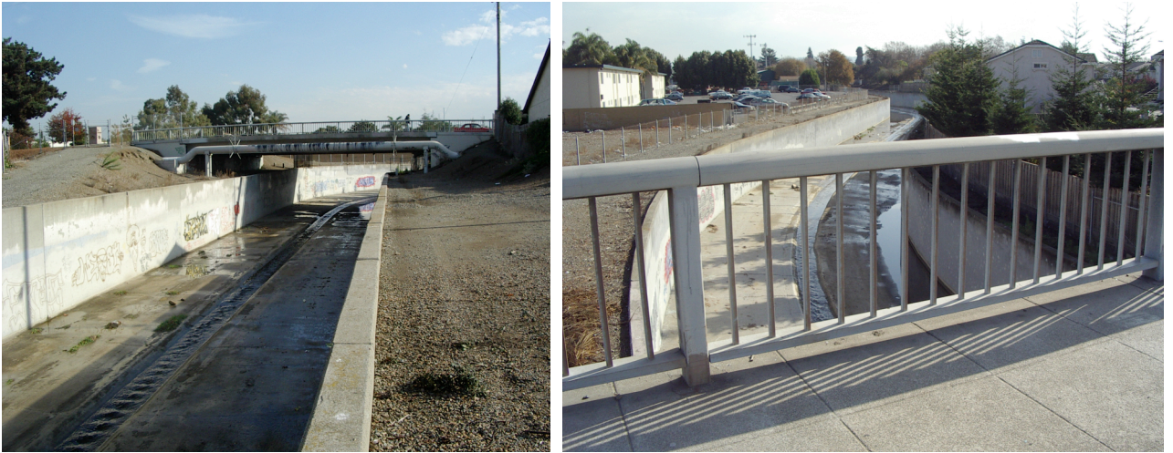
A) View looking upstream at the Washington Street Bridge. B) View looking upstream from the potential sample location on the upstream side of Washington Street.
