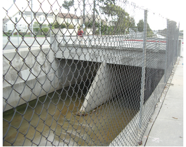
A) View looking upstream across West Orange Drive into Orange Memorial Park. B) Looking at the upstream side of the concrete double barrel culvert.
