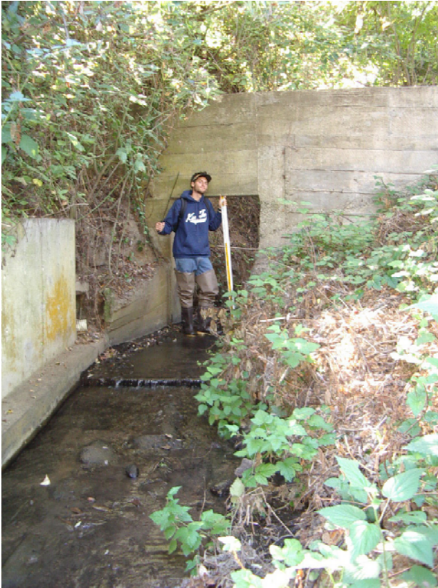
Figure 37. Photograph of concrete flashdam located on Sanchez fork, 669 ft (204) m upstream of the confluence.
