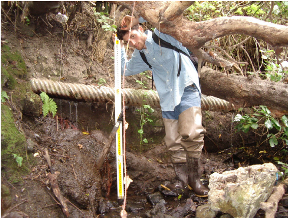
Figure 40. Photograph of failing culvert in Sanchez fork 1,316 ft (401 m) upstream of the confluence.
