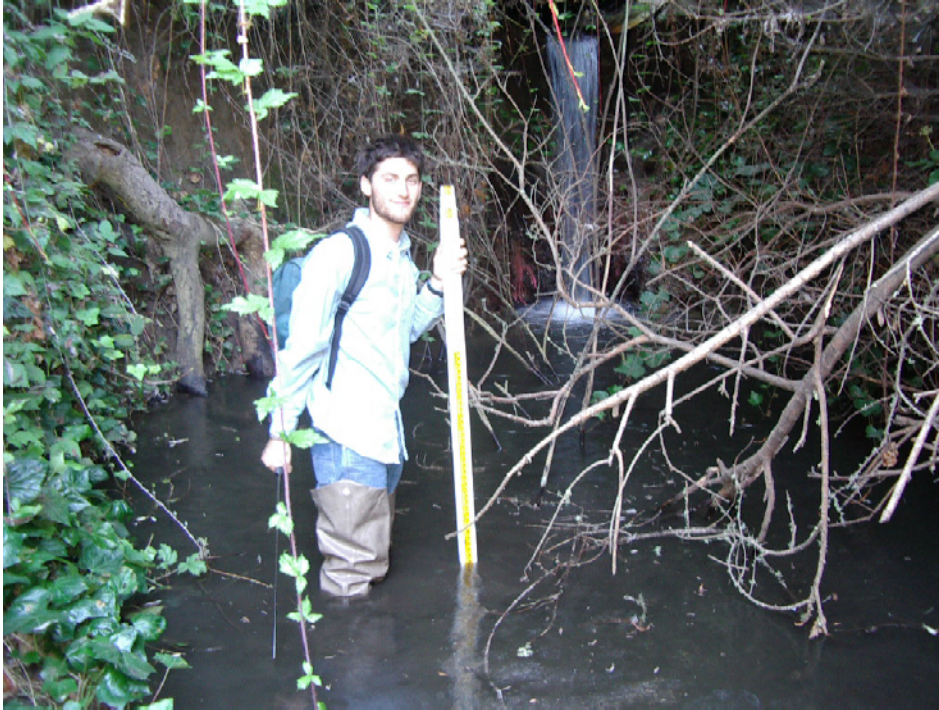
Figure 41. Photograph of the large culvert under the church parking lot and associated plunge pool in Sanchez fork, 984 ft (300 m) upstream of the confluence. This pool contains a large fine-grained pool deposit.
