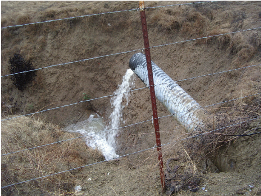
Figure 9. Photograph of the hanging culvert.
