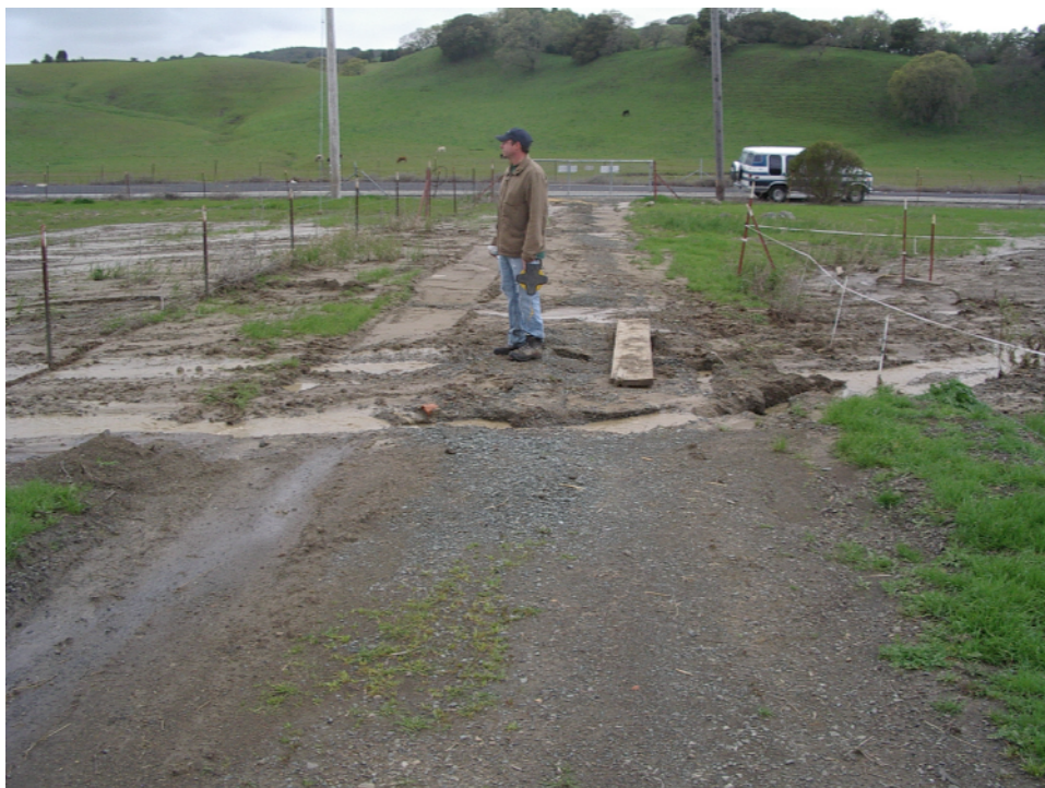
Figure 13. Photograph of clogged culvert, road erosion, and surrounding deposition of sediment on Gully C at the ranch road. Flow is from left to right.
