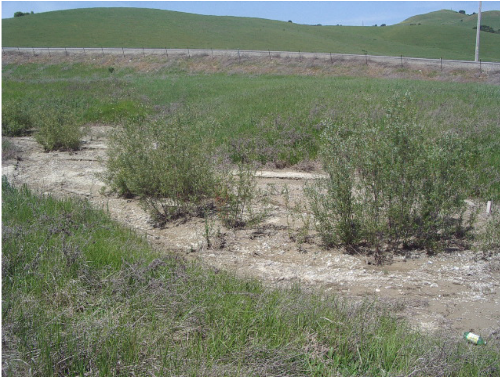
Figure 24. Photograph showing the aggradation that occurred at AXS4.
