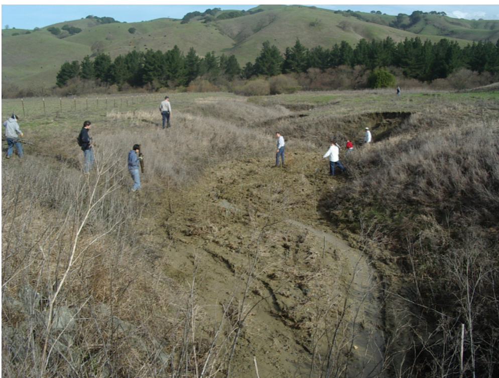
Figure A-34. Photograph of sediment deposition behind the check dam on Gully B. Photo taken looking downstream from the ranch road, during an EBMUD restoration day.
