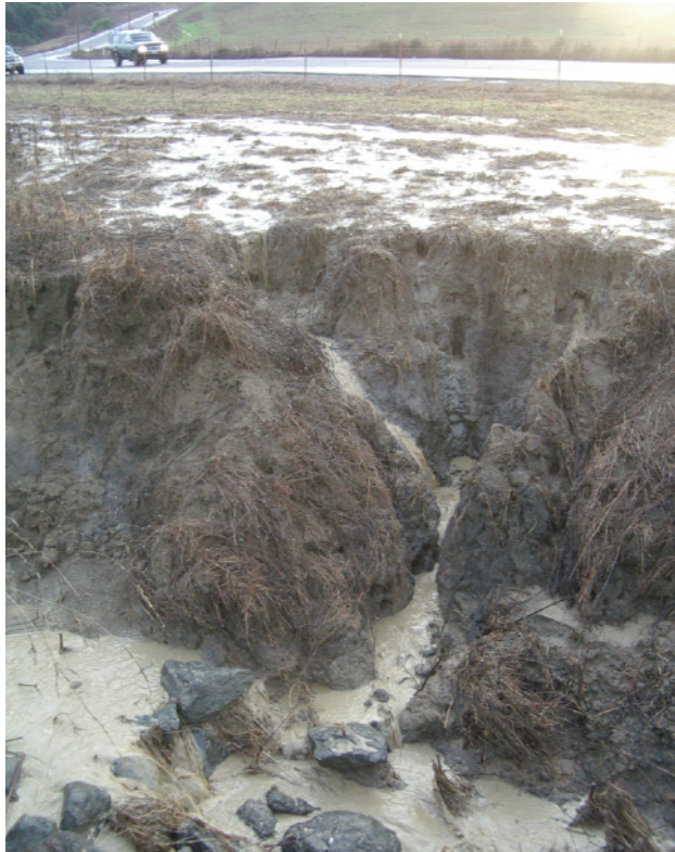
Figure A-72. Pasture surface flow returning into an incised reach of Gully C downstream of the ranch road, 1/2/2006.
