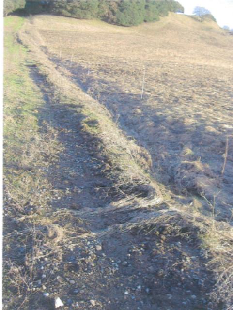
Surface runoff concentrating above access road, then flowing to eroded area below road. Gully D.
