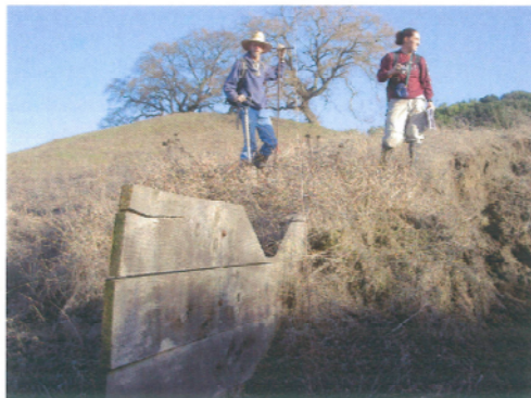
This check dam at Gully B was eroded around the side, causing further erosion impacts to the site.
