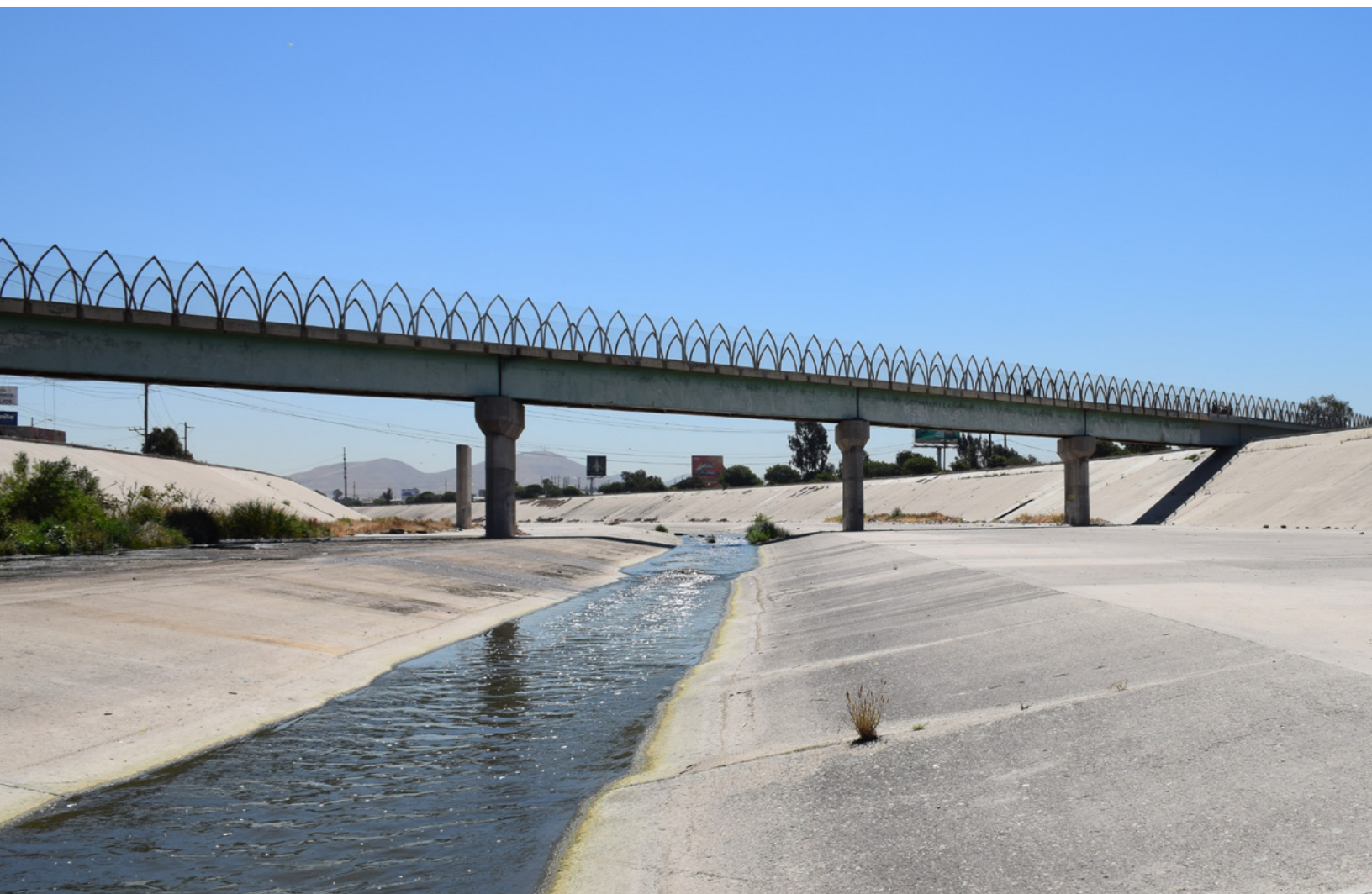
Figure 7.14. A concrete trapezoidal flood control channel , completed in 1979, carries flows from downstream of Matanuco Canyon to the international border. It is seen here beneath the railroad bridge near the former site of the Agua Caliente hot springs. (Photo by Samuel Safran, April 2015)
