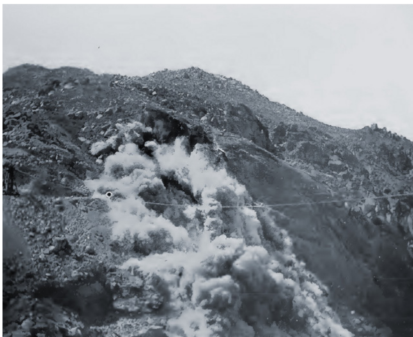
Figure 3.21. "Explosion at Morena dam site," December 26, 1896. Rock used to construct Morena dam was obtained from the adjacent hillsides. This photograph, taken December 26, 1896, shows an explosion at the dam site that reportedly dislodged 200,000 tons (200 million kg) of rock. (Newell 1901, Part IV, Pl. LV, courtesy Internet Archive)
