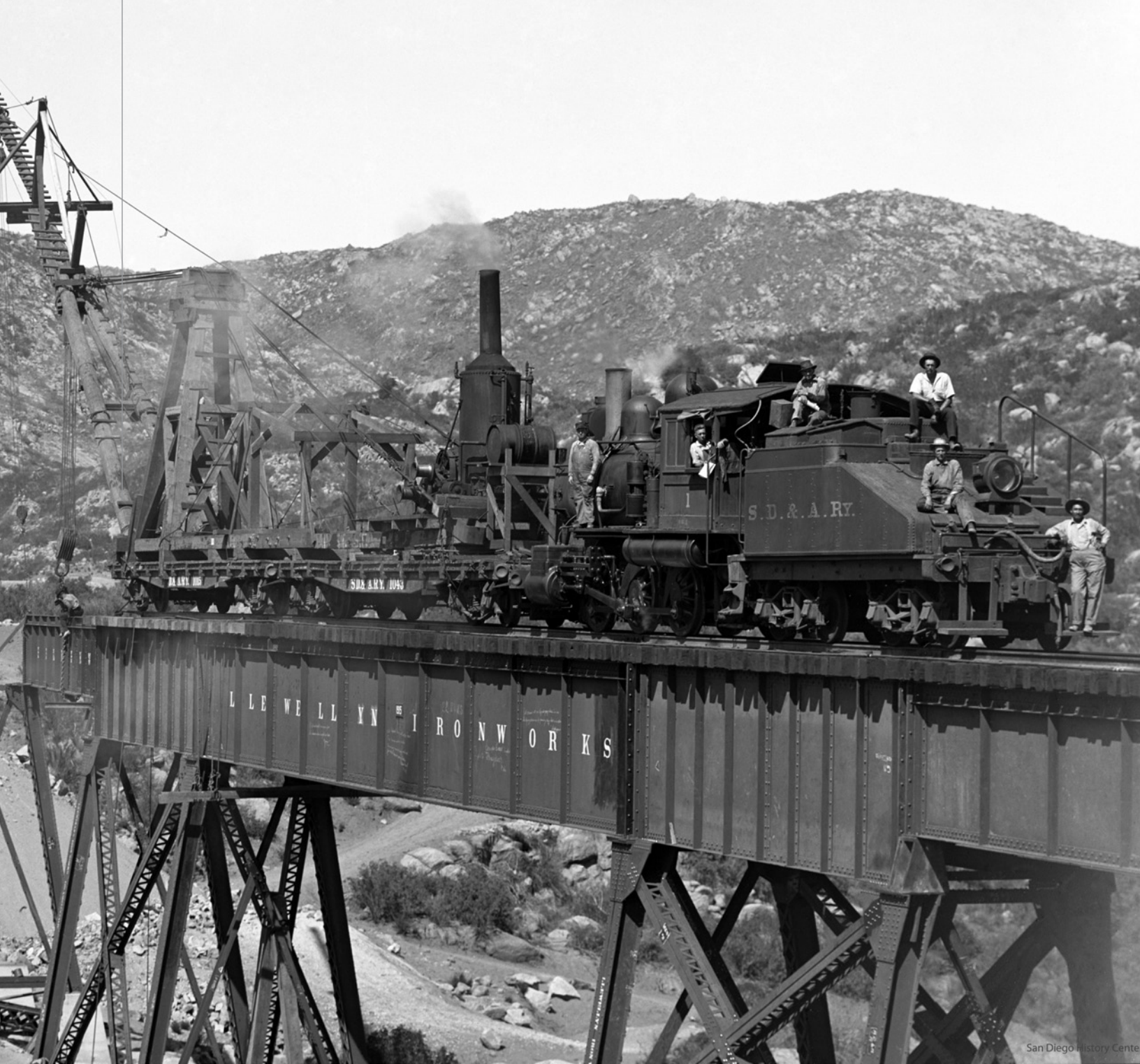
Figure 3.8. Construction of the San Diego-Arizona Eastern Railroad trestle over the Tijuana River across Matanuco Canyon, ca. 1910. (Photo #7717, courtesy San Diego History Center)
