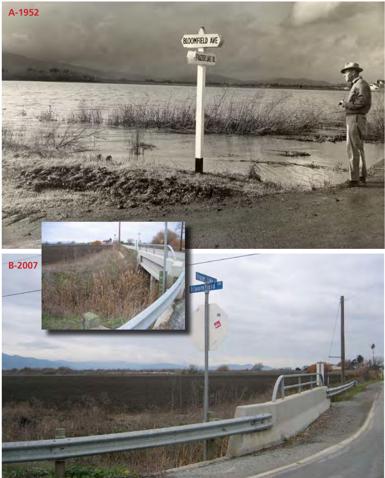
Figure 5.4. The former wet meadows east of Llagas Creek, flooded in February 1952 (A) and the same site in 2007 (B). Modifications to reduce overflow (inset) include drainage channel (note cattails in foreground), culvert under bridge crossing, and raised roadway. (A: Unknown 1952, courtesy of the Gilroy Museum)
