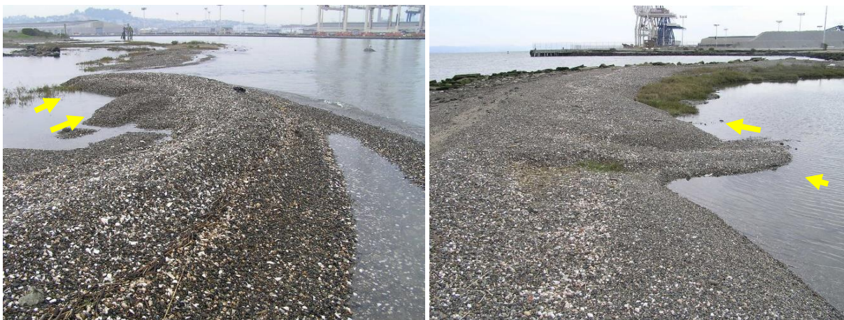
Figure 6. Rapid wave-reworking of coarse beach sediments occurred along the outer northern shore of Pier 94 during the first winter after beach sediment nourishment. Multiple recurved spits at open breaches and inlets (arrow), and relict recurves where tidal passes were aggraded and closed, indicate rapid longshore drift, predominantly to the northwest. February and March 2006.
