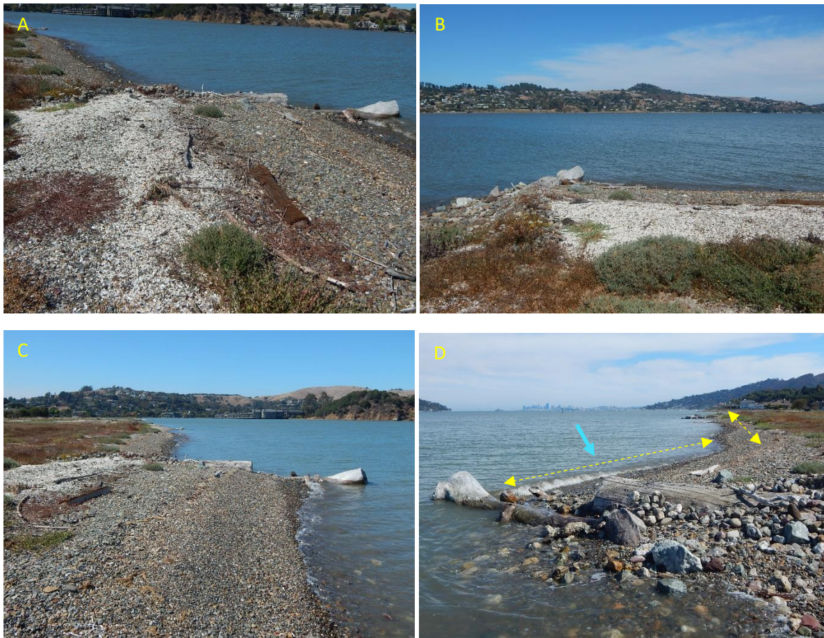
Figure 10. Short groins ("micro-groins", or drift-sills of embedded, pinned logs and boulders) along the Central littoral cell of Aramburu Island trap updrift accretion wedges of coarse sediment that prograde seaward, a characteristic of drift-aligned beaches (A-C). Downdrift sides of groins either remain stable or exhibit erosion where drift of beach sediment is obstructed locally. When gravel beach profiles retreated landward over time, beach accretion wedges on the updrift side of groins reorient to face dominant wave approach (D), in contrast with the strongly oblique orientation of the main beach axis relative to wave approach.
