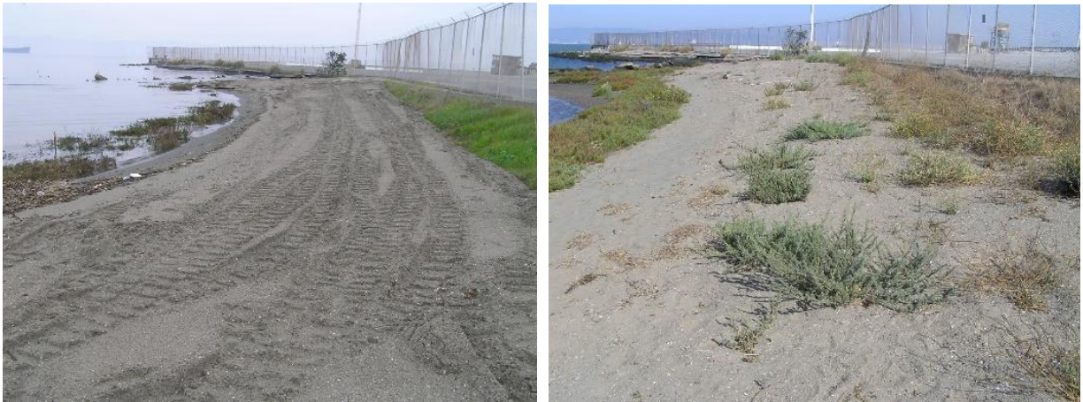
Figure 34. The south shore of Pier 94 a month after construction (left, Feb- 2006) and after initial planting with the endangered estuarine beach/salt marsh shrub, California sea-blite in March (Sept 2006), exhibiting a full beach profile above a low tide terrace fringed with pickleweed salt marsh (Fig 36).
