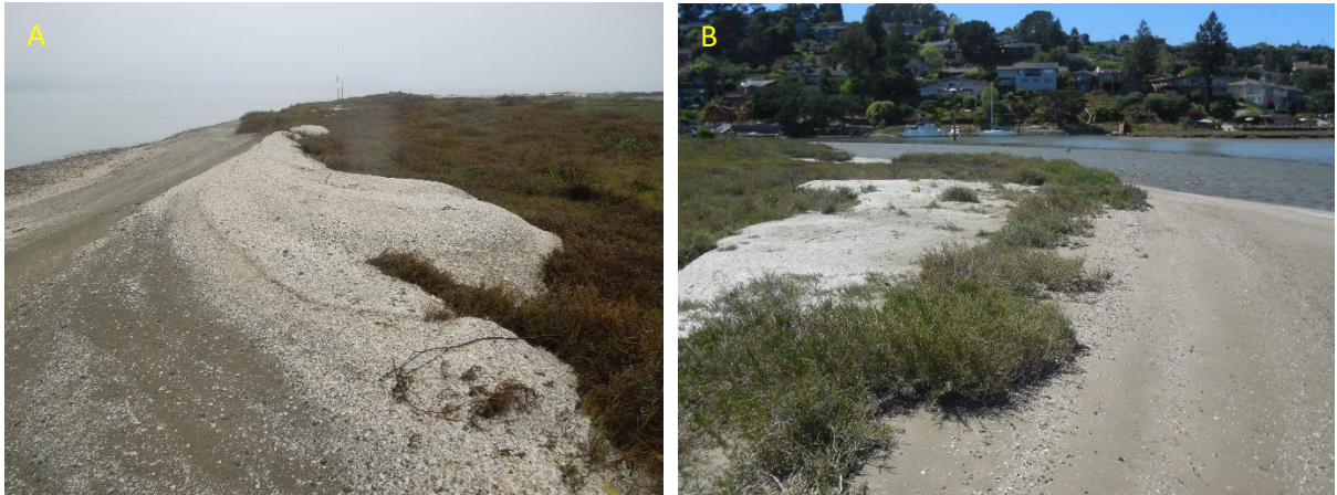
Figure 31. Initial beach progradation at the edge of salt marsh along the north end of Aramburu Island down-drift of beach nourishment areas, December 2012 (A, post-construction drift) and April 2013 (B, ongoing drift), along pre-project salt marsh erosion scarps. Sand was deposited both on top of salt marsh (pickleweed) vegetation landward of the previously erosional marsh edge, and bayward of the marsh, on mudflats.
