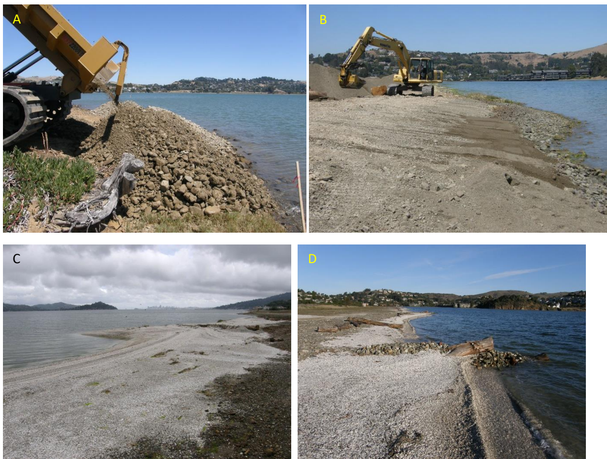
Figure 14. Rapid complete wave-reworking of coarse beach sediment placed at Aramburu Island, central shoreline. (A-B) Engineered placement of all beach sediment (cobble, gravel, sand and shell hash) across the upper intertidal profile, August 2011. (C) High tides and waves overtopped new beach fills, concentrating lighter oyster shell hash in newly wave-deposited beachfaces and berm tops with natural morphology. Most original graded surfaces and fills are eliminated within 2 months; minor vehicle tracks persist. October 4, 2011. (D) Micro-groins rapidly develop updrift/downdrift asymmetry due to updrift accretion of gravel and shell hash, eliminating original beach fill grading and vehicle track patterns. December 22, 2011.
