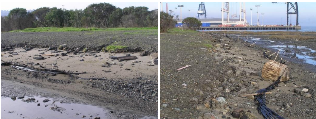
Figure 3. Severe storm wave erosion of the interior north shore of Pier 94 occurred during the New Years 2006 storms (immediately prior to beach nourishment) in the absence significant wave-sheltering by outer barrier beaches. January 6, 2006.
