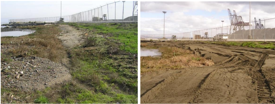
Figure 4. Pre-project shoreline conditions at the south shore of Pier 94 (left, January 5 2006), and post-grading beach sediment nourishment (right; January 26 2006), adding to pre-existing sand and gravel derived from local erosion, and occasional runoff from the adjacent sand import offloading facility.
