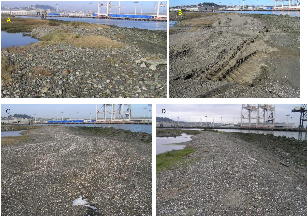
Figure 13. Rapid wave reworking of poorly sorted sand, gravel, and shell sediment (dredged bay sand, non-commercial screenings from sand refining) at Pier 94 north shore, Port of San Francisco. (A) Pre-project shore platform composed of decomposing concrete rubble and debris (lag armor), with patchy high salt marsh vegetation, January 6, 2006. (B) Nourished beach sediment placed by small ground-based equipment (bobcat), January 23, 2006. (C) Multiple natural gravel and sand beach ridge landforms deposited after winter storm wave reworking of placed sediment; minor residual of vehicle tracks. February 6, 2006. (D) Complete reworking of coarse beach sediment to single gravel storm berm by November 16, 2006.
