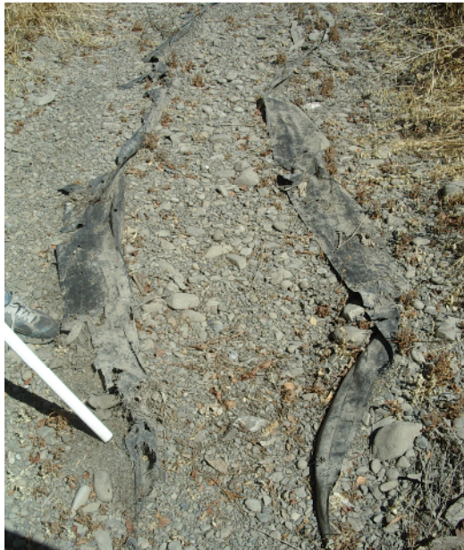
Appendix Figure 23. Photographs of gabions armoring the Dry Creek flood control channel. Upper left: photo showing exposed bank gabion. Upper right: photograph showing gabions on the bed surface. Lower left: exposed erosion control fabric. Lower right: exposed bed gabion.
