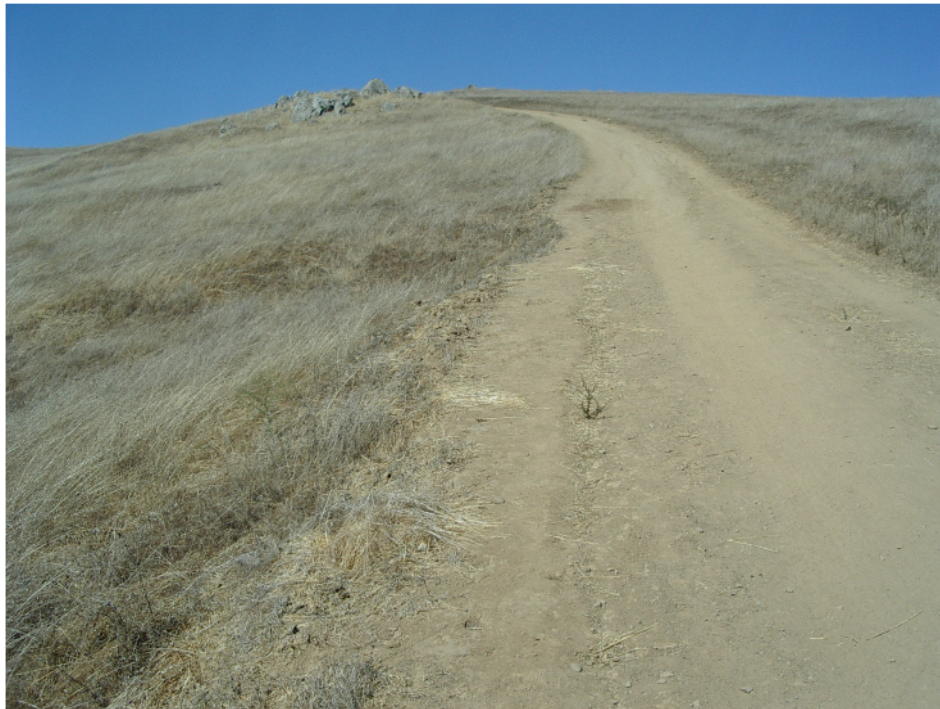
Appendix Figure 14. Photograph looking uphill at a road segment contributing to erosion; runoff exits the road to the left (middle of the photograph), and has contributed to the destabilization of the hillslope.
