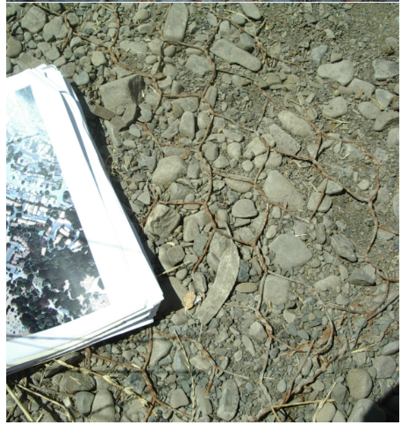
Appendix Figure 23. Photographs of gabions armoring the Dry Creek flood control channel. Upper left: photo showing exposed bank gabion. Upper right: photograph showing gabions on the bed surface. Lower left: exposed erosion control fabric. Lower right: exposed bed gabion.
