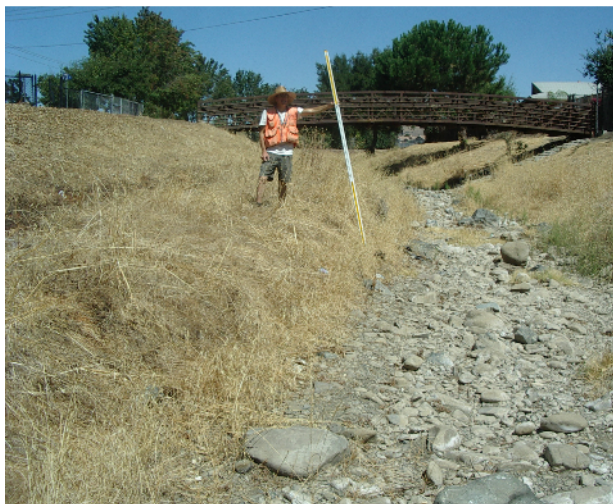
Appendix Figure 20. Left: Photograph showing a package of sediment deposited within the flood control channel. Right: a close-up of the heterogeneous nature of the deposit.
