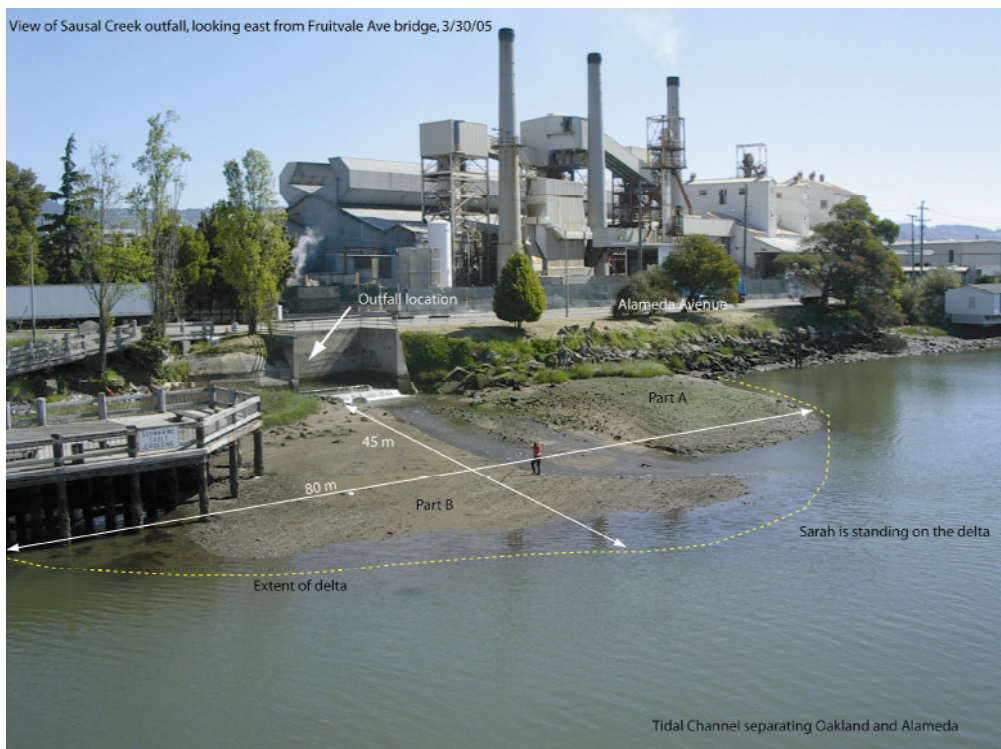
Figure 3. Sausal Creek outfall Delta located near the Fruitvale Avenue Bridge to Alameda. Note the prominent delta impinging on the shipping channel at this location.
