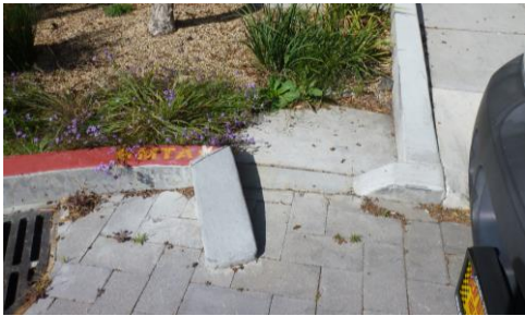
Figure 15. One of the two curb extensions added in December 2012 to better direct runoff into the bioretention planter.
