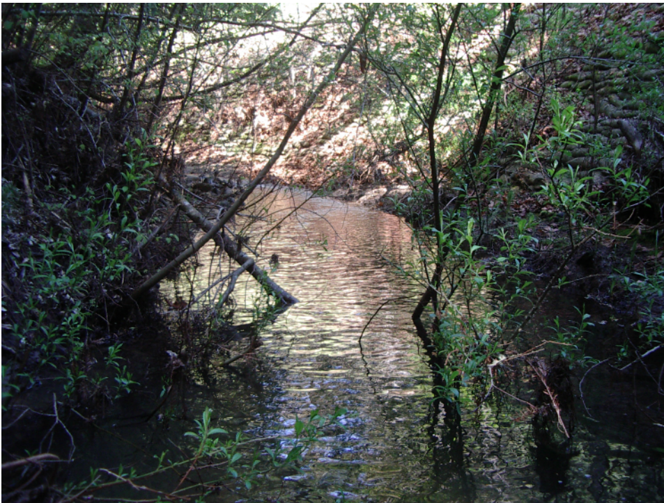
Figure 37. Channel bank revetment (sacrete) along the outside of a meander bend in reach 3A (S. Pearce, 2007).
