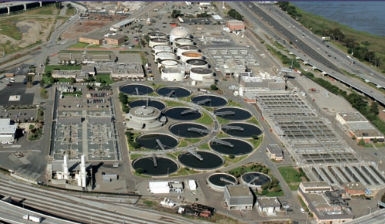
East Bay Municipal Utility District wastewater treatment plant. Photograph by Greg Keller.
