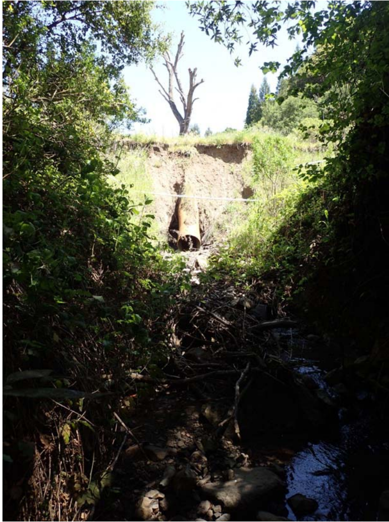
Figure 40. Field photograph looking upstream at the knickpoint (labeled 4.95m high knickpoint in Figure 39) and collapsed culvert.
