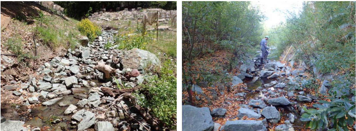
Figure 26. Illustration of the large grain size of the placed rock within the channel.
