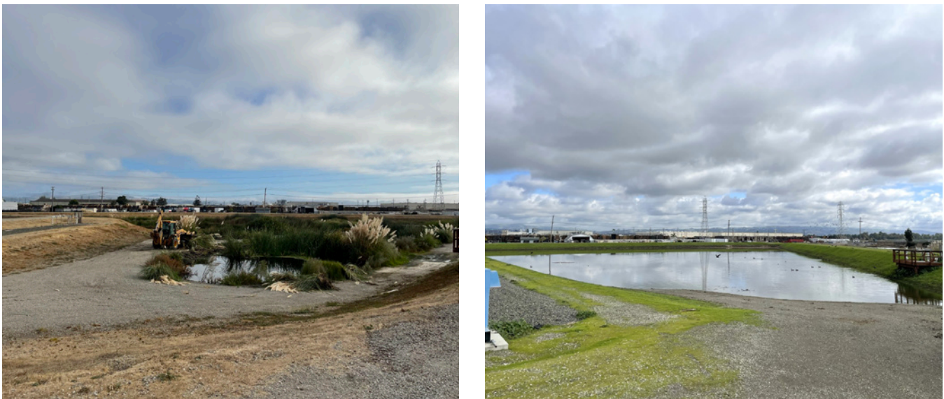
Figure 1. The wet weather FEB at Oro Loma Sanitary District, which was historically used as a pilot open-water wetland for pre-treatment. Left: summer condition (open water wetland). Right: winter wet weather storage. Photos by Ellen Plane, SFEI.
