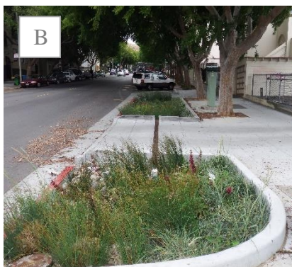
Figure 1. A) Locations of seven monitored planters within the Cesar Chavez Streetscape Improvement Project. B) View of the Folsom Street SW bioretention planter in dry conditions, and C) under storm conditions.
