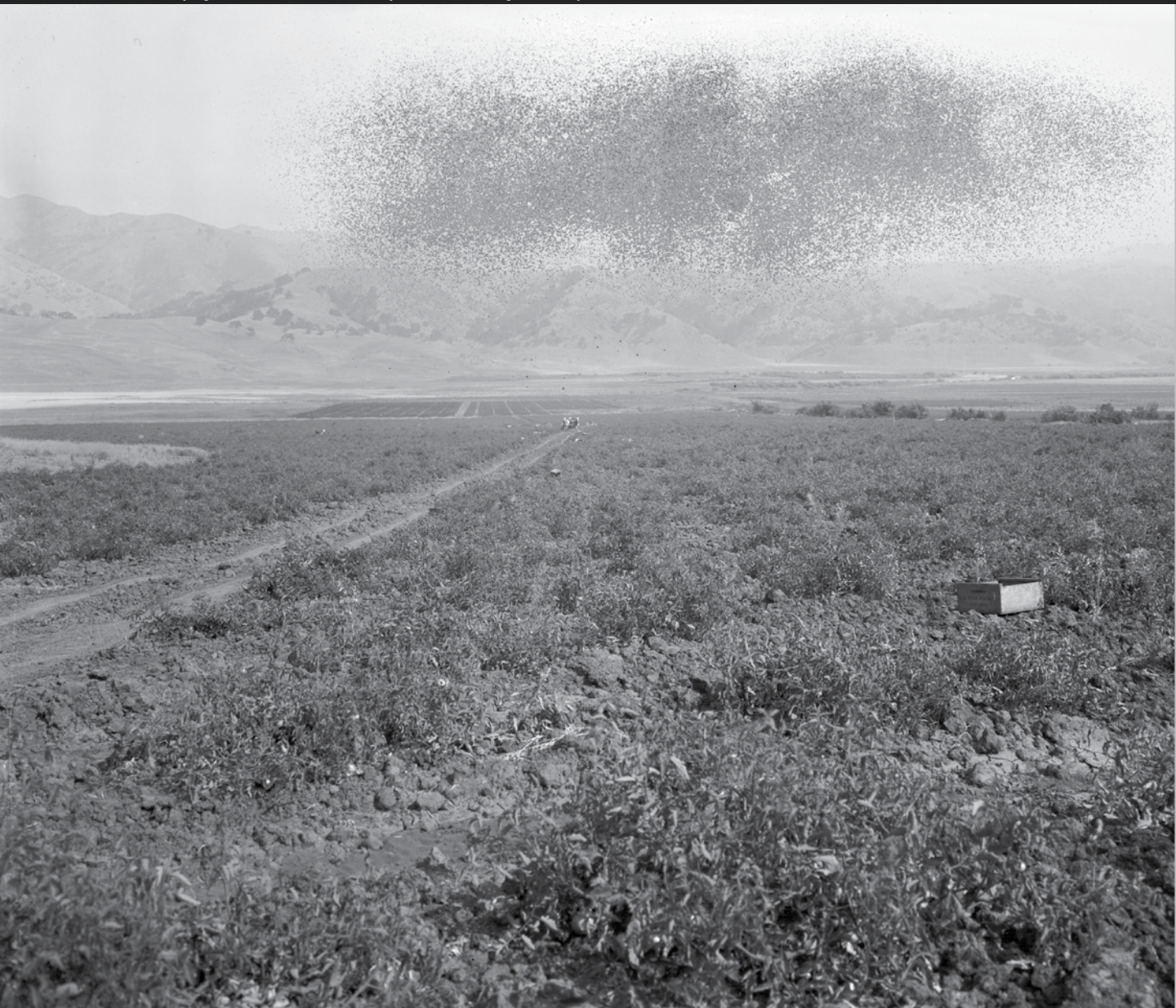
Early agriculture in Calaveras Valley, 1919. (D-92, image courtesy of the San Francisco Public Utilities Commission)
