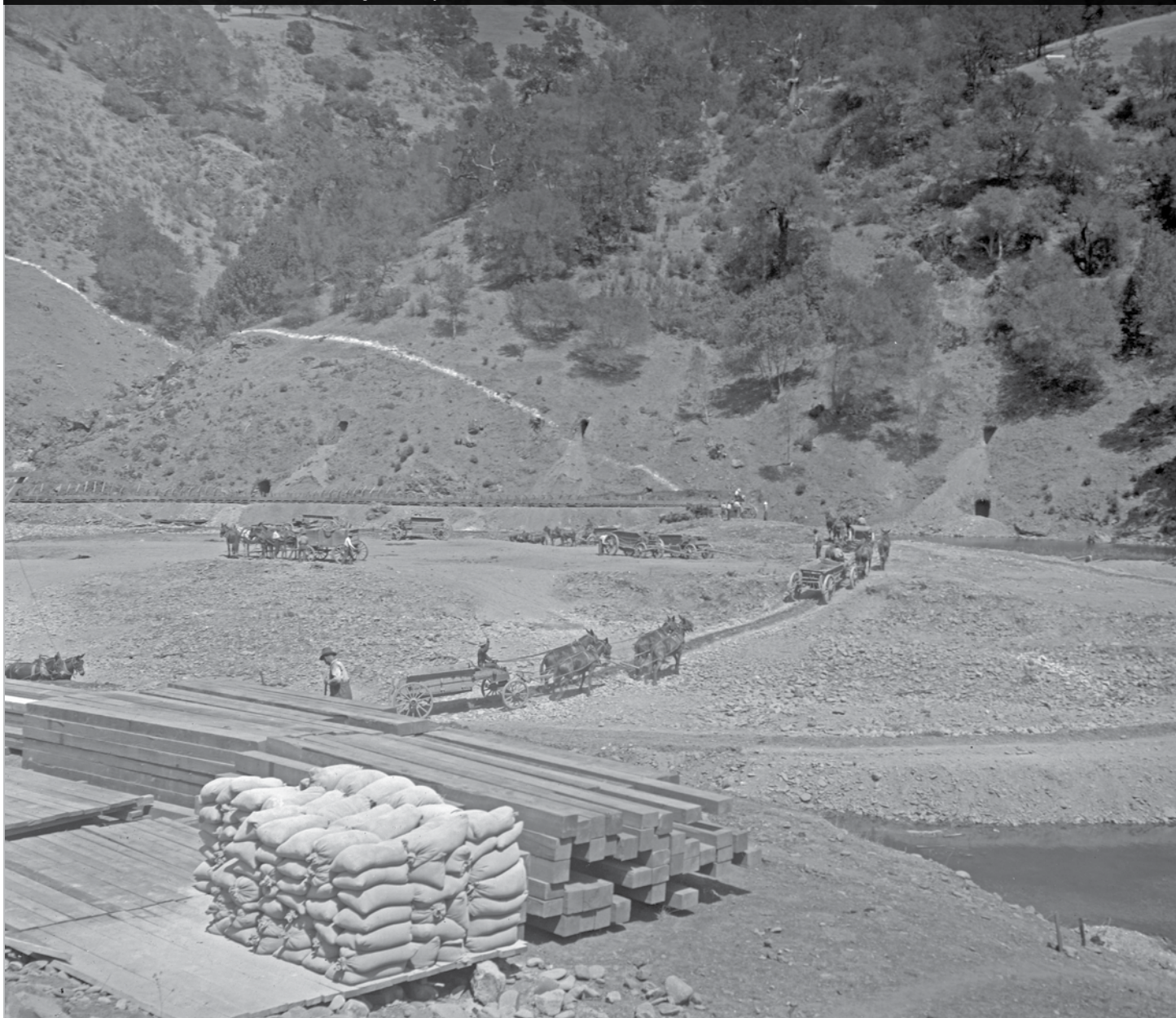
Construction of Calaveras Dam, 1913. (C-312, image courtesy of the San Francisco Public Utilities Commission)
