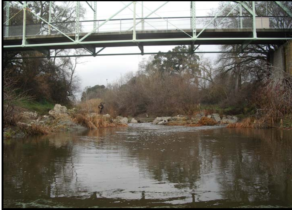
Figure 74. Looking upstream at the riprap and old bridge footer debris that is stabilizing the bed elevation at the Verona bridge.
