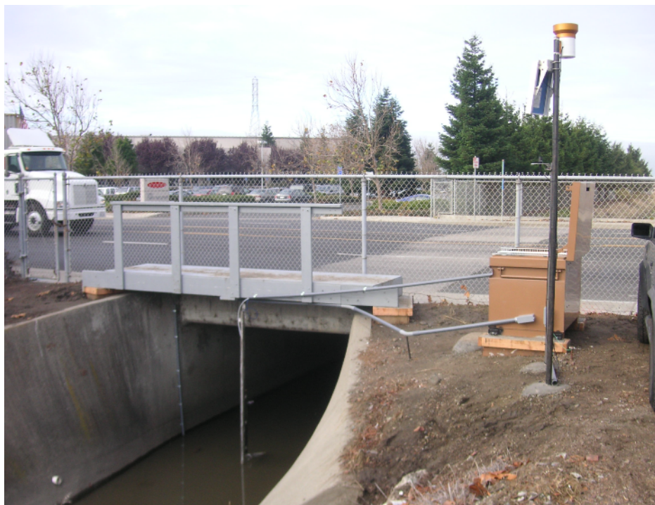
Figure 11. The instrumentation set-up at Zone 4 Line A, including the metal box housing the ISCO pumping sampler, datalogger and battery, the wooden sampling platform, the sampling boom, solar panel and tipping-bucket rain gauge.
