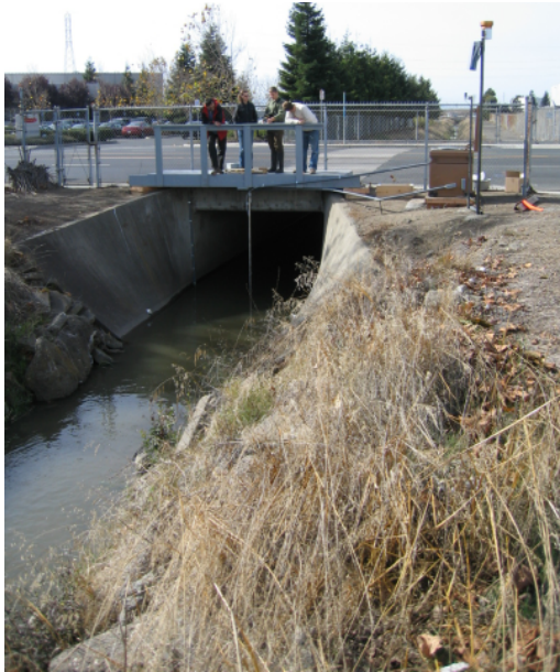
Figure 6. Single-barrel box culvert. Figure 7. Cross-section of channel at sampling location.
