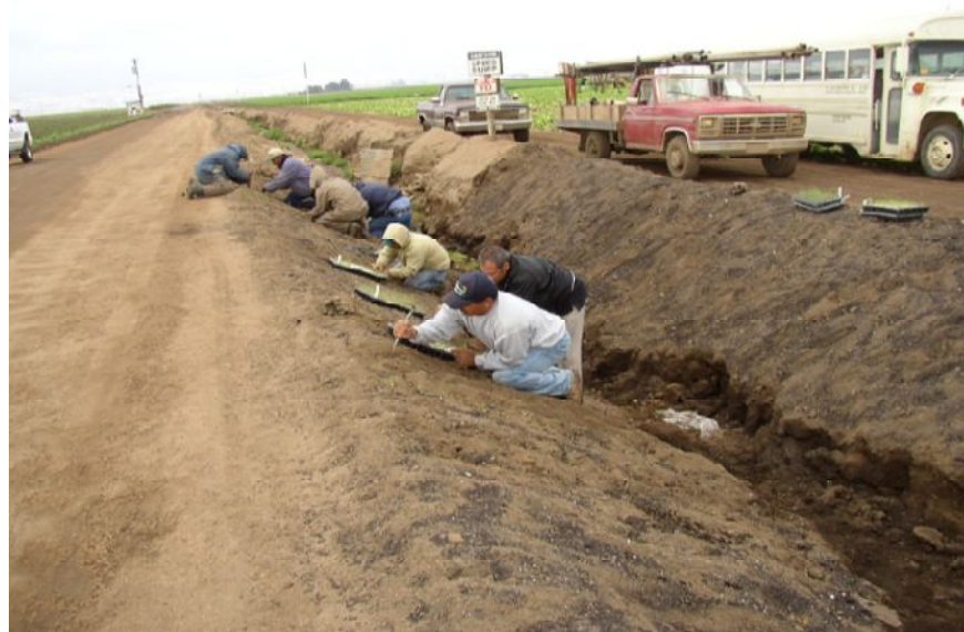
Figure 7. Planting grass plugs, one at a time.
