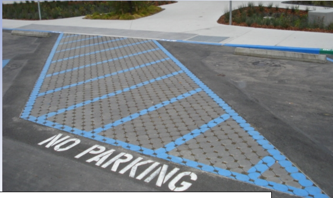
Small area of pervious pavers, Serramonte Library
