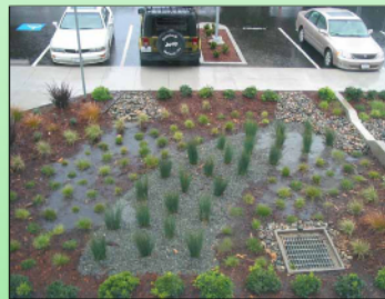
During very heavy storms, runoff ponds up and eventually overflows into the storm drain inlet to prevent flooding.
