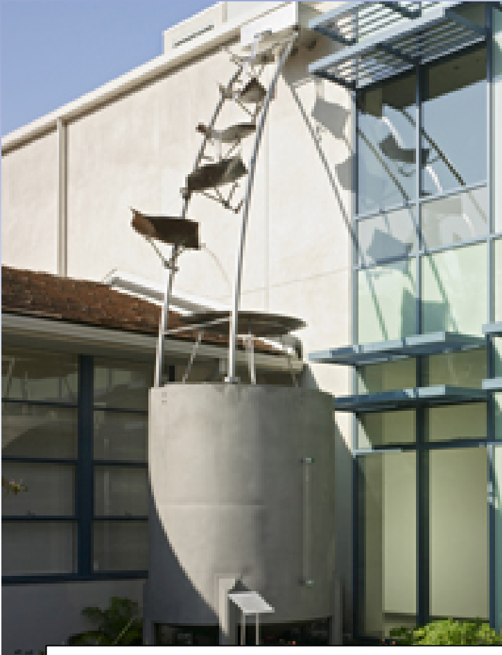
Sculpture collects rainwater for flushing toilets, Mills College Natural Sciences Building, Oakland
