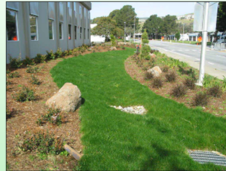
The bioswale along Valley Drive also collects and treats stormwater runoff.
