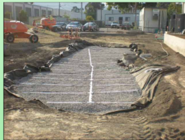
The underdrain system beneath the rain garden carries treated stormwater runoff to the Brisbane Lagoon and out to the Bay.
