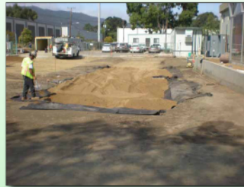
The rain garden uses a special soil mixture to help runoff soak into the ground and plants that do well in wet conditions.
