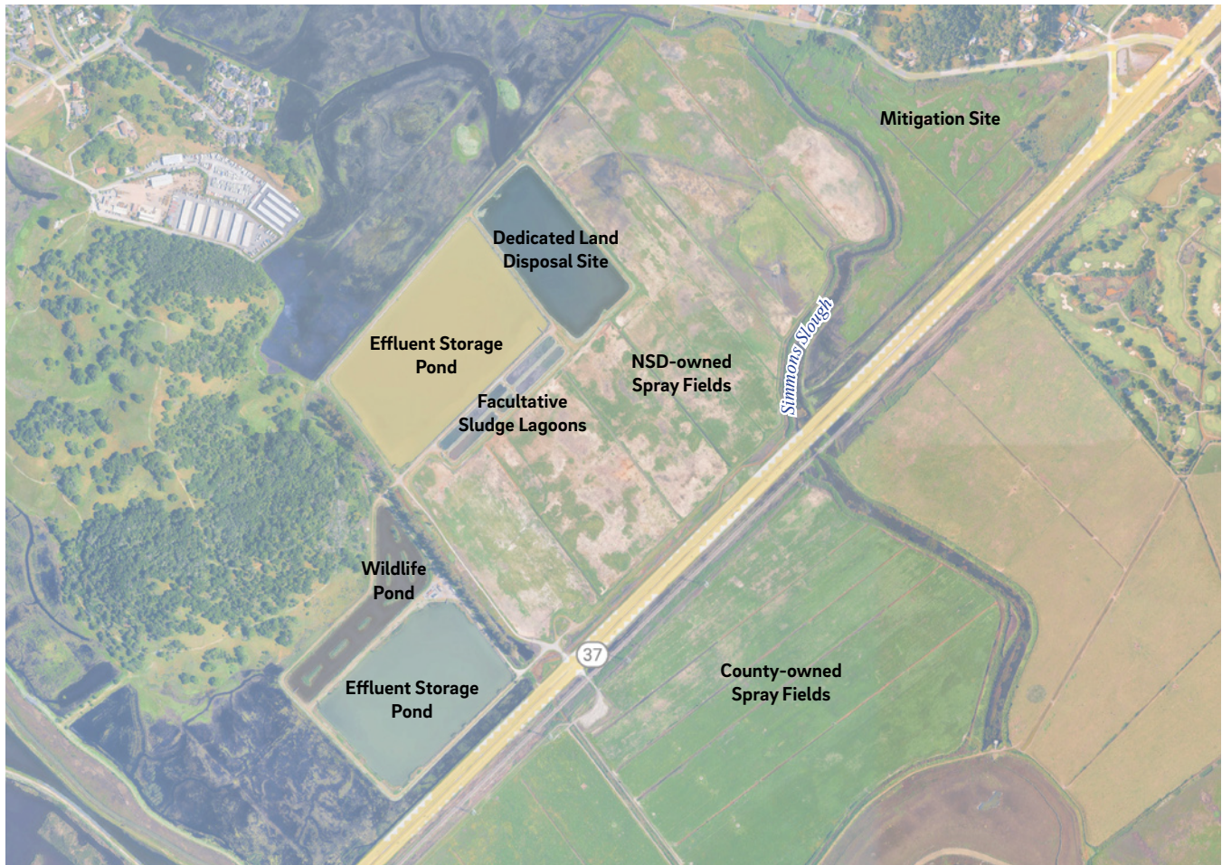
Figure 4.16. Novato Sanitary District infrastructure in the Simmons Slough area.
