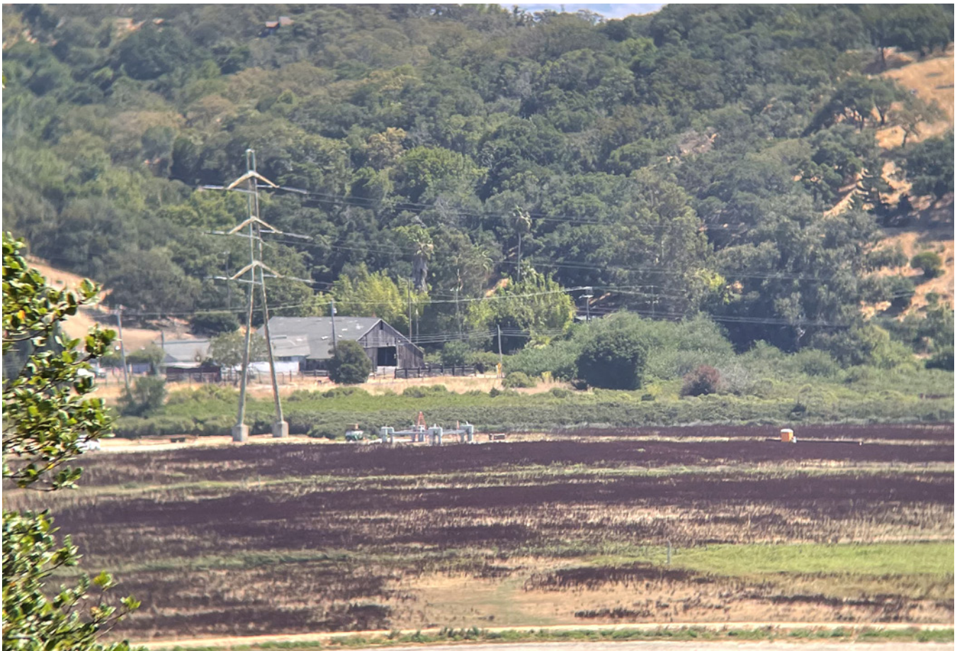
Electric transmission tower foundation replacement underway in NSD sprayfields near Simmons Slough, August 2025. Photo by Ellen Plane, SFEI.
