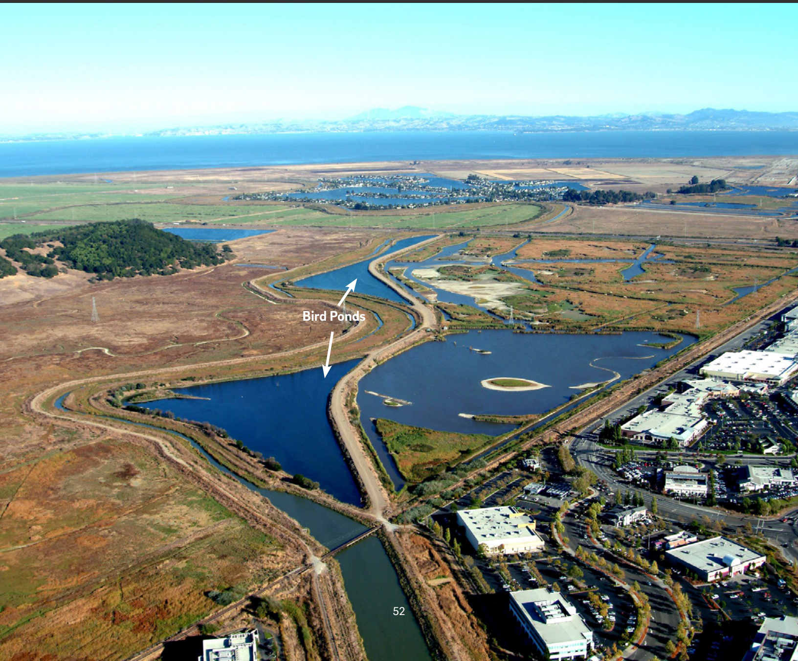
Aerial view of the Novato baylands, looking downstream over the Bird Ponds toward San Pablo Bay. Photo by Sue Lattanzio.
