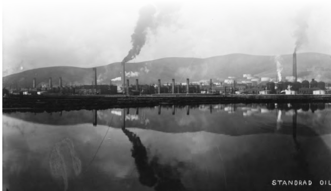
Early industry at the edge of the Bay. The Standard Oil refinery at Point Richmond, 1910. (Courtesy of the Richmond Public Library)
